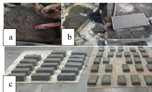
Gambar 3. Mix Design Paving Block Variasi
